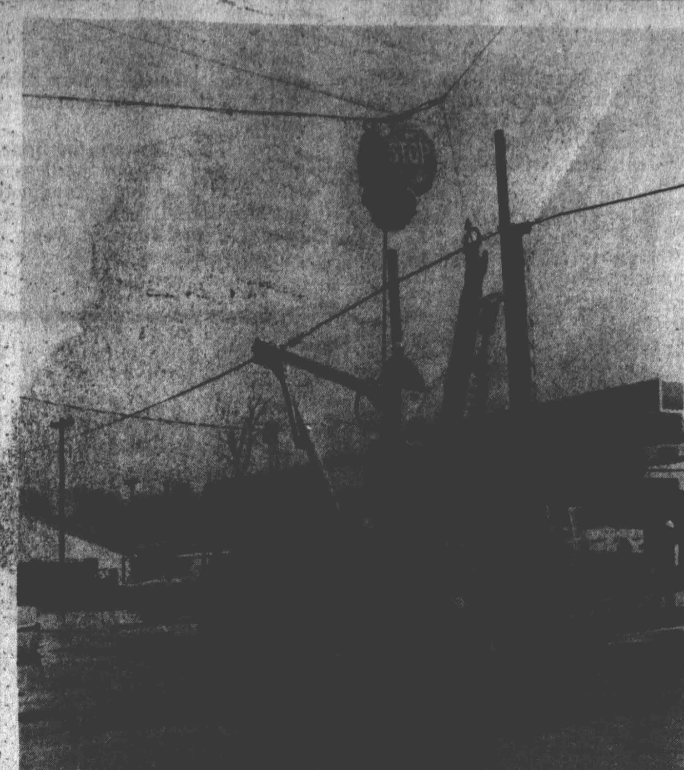
STOP-AND-GO TRAFFIC LIGHT at Church and Tigrett in Halls was raised Thursday of last week to the required 17 feet after Ripley Power & Light changed poles in front of Key Corner Exxon.
